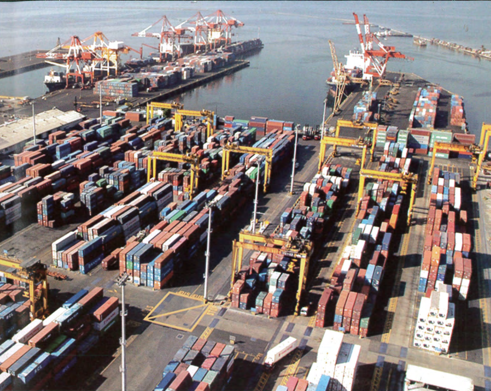
Photo courtesy of ATI
