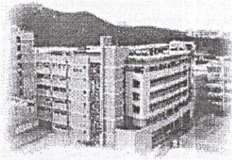
Whole view of GSPA Bldg. 57-1
